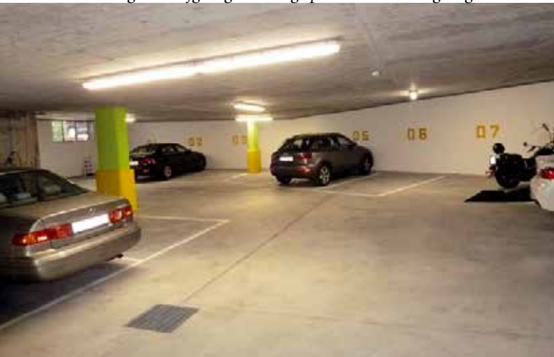
hoteleigene Tiefgarage / Garage privato / Private garage
